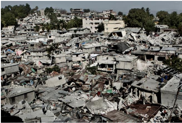
Figure #1: 2010 Haiti Earthquake
